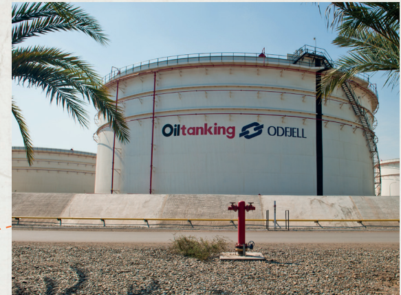
Oiltanking Odfjell Terminals (Oman)
