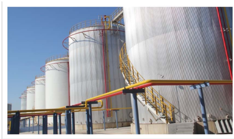
New tank farm at the Tianjin Terminal in China
