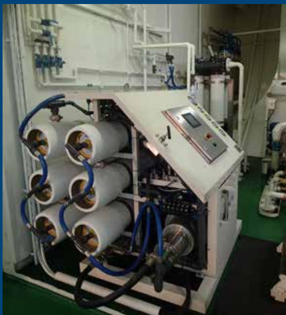
Reverse osmosis plants will be installed on 26 vessels to reduce boiler consumption
